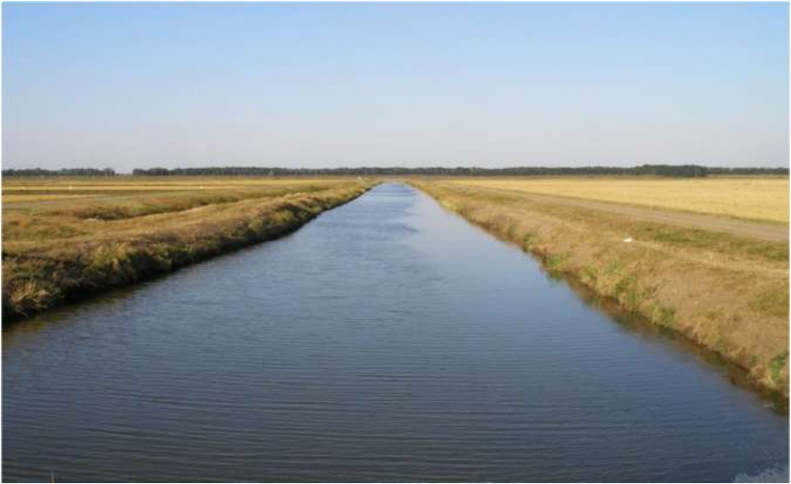
Figure 64 – Main Irrigation Channel
