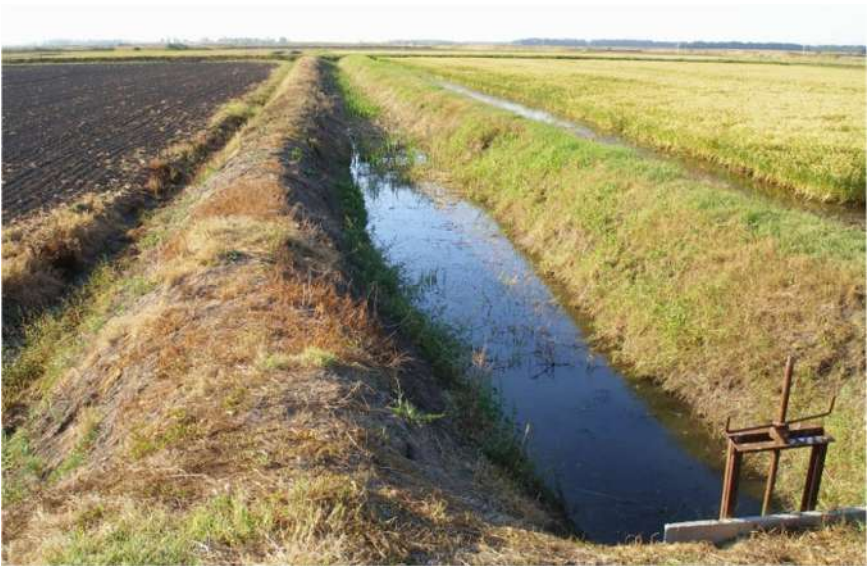
Figure 65 – The field irrigation canal with hydraulic engineering installations
