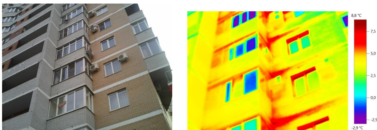
Fig.2 – Fragment of the facade of a building not equipped with a ventilated facade
